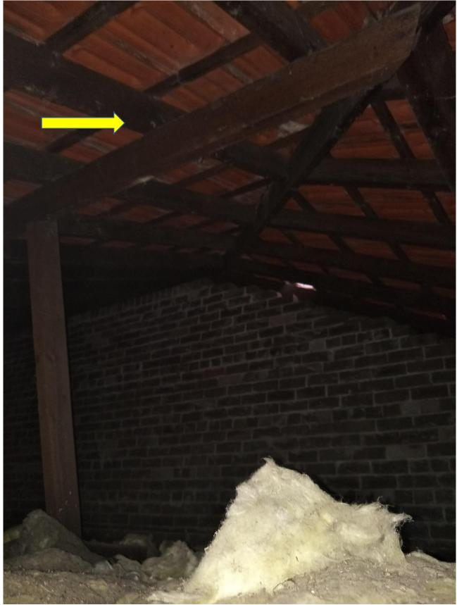
Figure 5no evidence of sarking observed in the roof, this is common with homes of this era.
