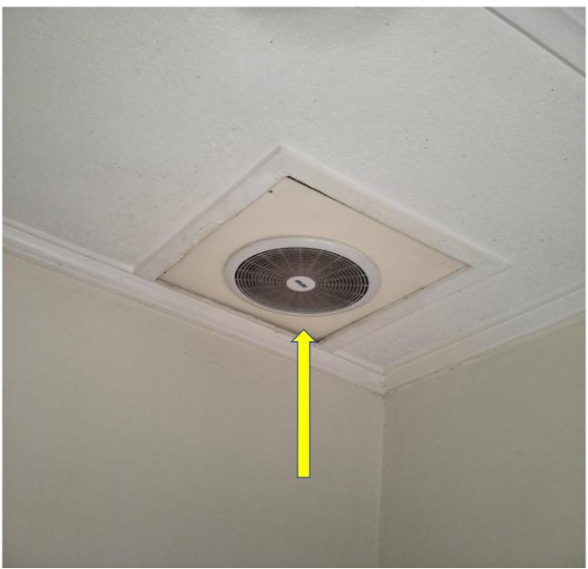
Figure 4the man hole has an electrical fan in which is a safety hazard. This should be moved into a new location. Engage a licenced electrician to attend to this.
