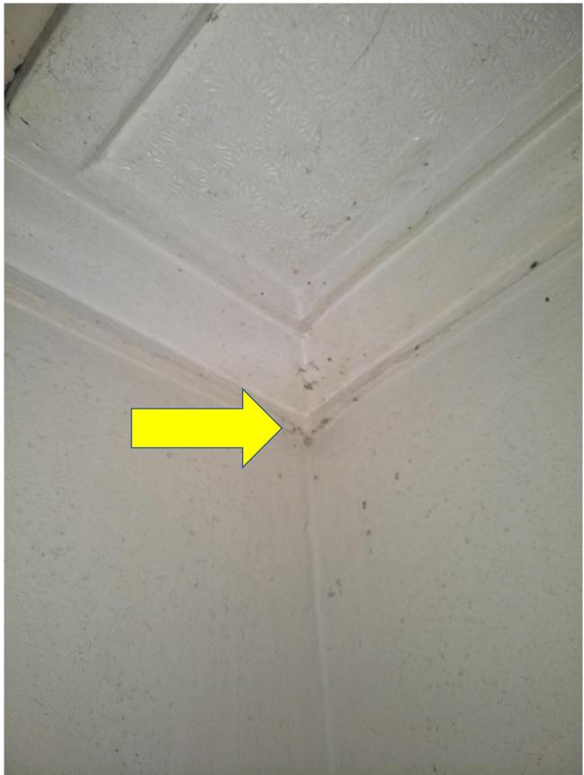
Figure 7evidence of mould located in the shower location due to inadequate ventilation.
