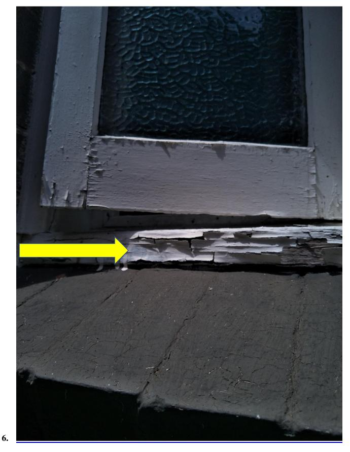
Figure 12 timber work around windows is in a dilapidated state.
