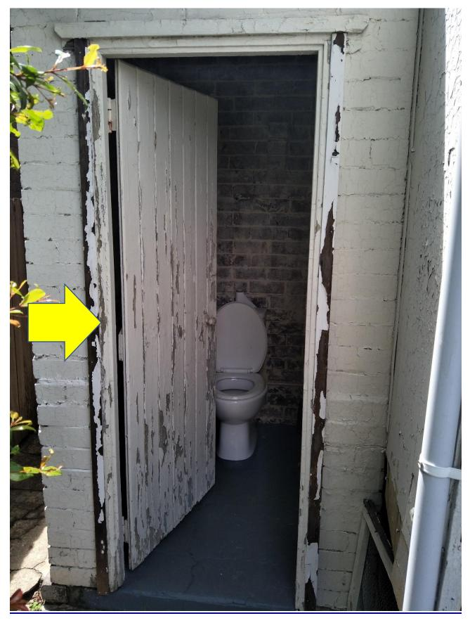
Figure 10timber work around the house requires painting and maintenance. Engage a carpenter and painting contractor to rectify.
