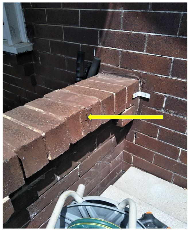
$Figure\ 2\ brick\ work\ exterior\ front\ has\ been\ repaired\ and\ requires\ relaying\ bricks\ by\ a\ licenced\ brick\ layer.$
