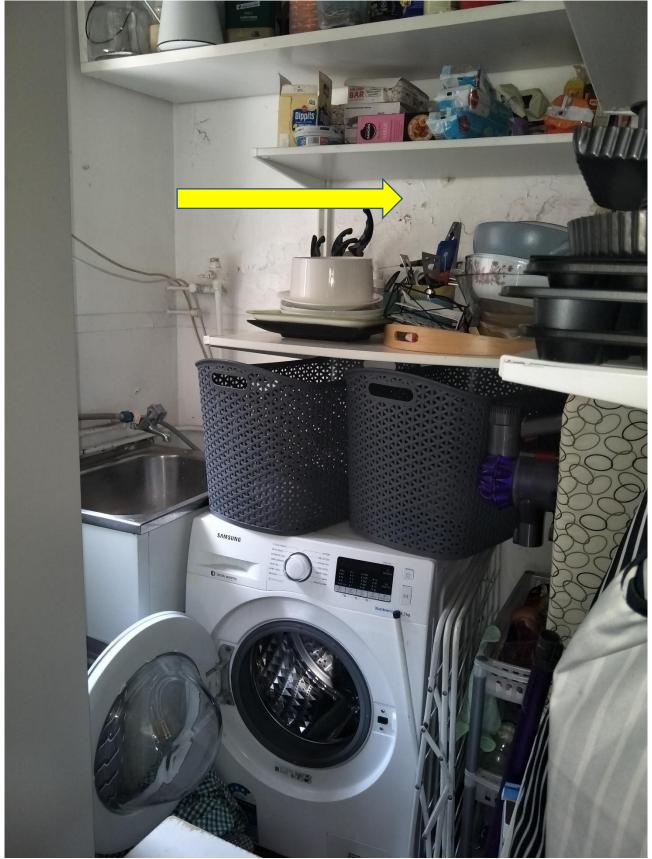
Figure 9the walls to the laundry have evidence of water ingress from the shower located directly adjacent to the location.
