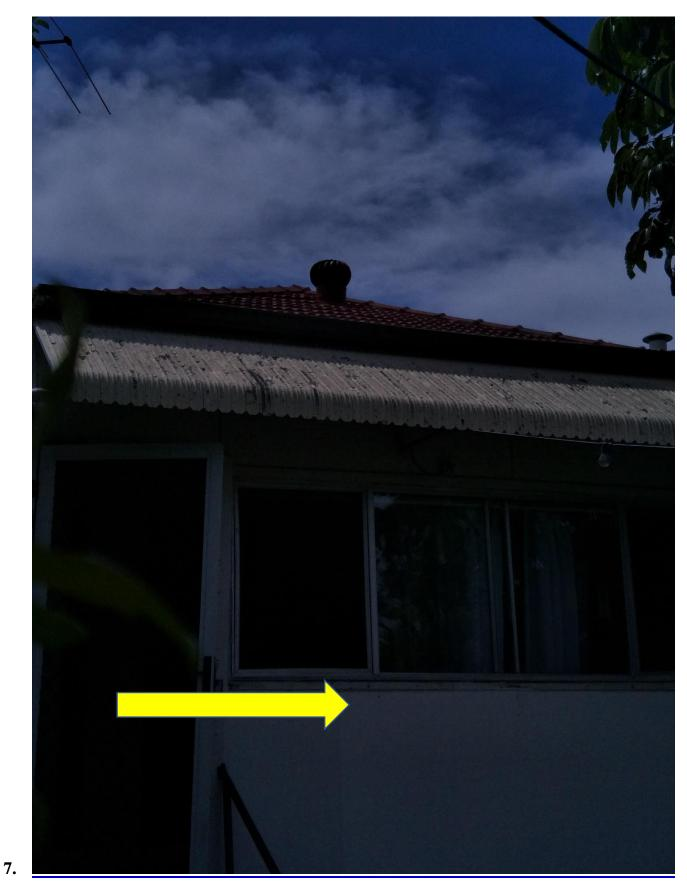
Figure 13the rear panel has evidence of possible asbestos on the rear wall lining this requires further testing.
