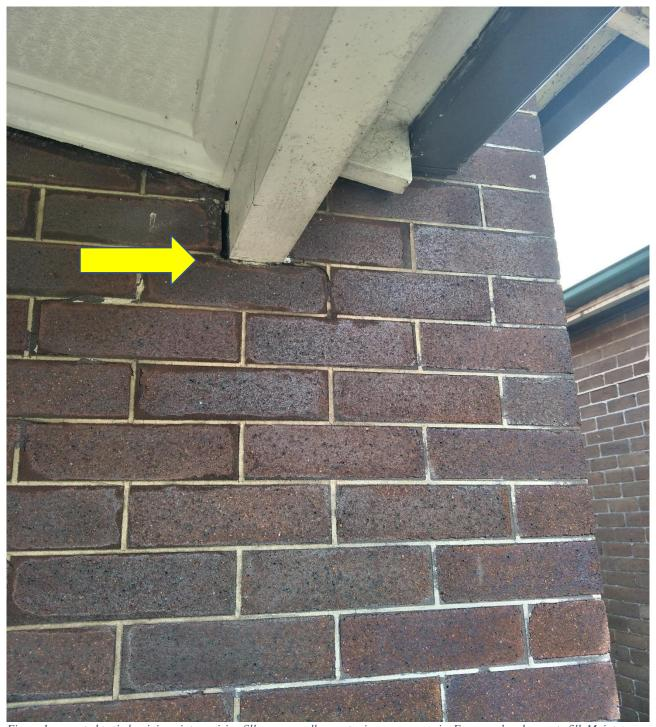
Figure 1 gap noted to timber join point requiring filler as may allow water ingress or vermin. Engage a handy man to fill. Maintenance defect.
