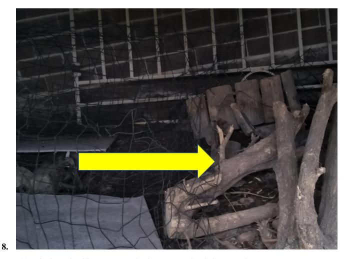
$Figure\ 14 stored\ timbers\ in\ the\ subfloor\ require\ removal\ as\ this\ may\ increase\ the\ risk\ of\ termite\ attack.$
