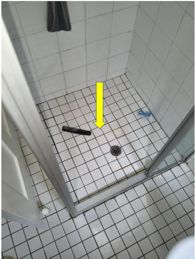
Figure 3the shower recess requires grouting, Engage a handy man to apply new grout.
