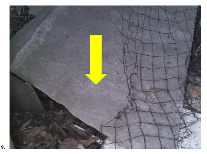
Figure 15 material that appears to be asbestos is found in the subfloor making it a safety risk to crawls where there may be asbestos, it is recommended the asbestos be removed and disposed of.
